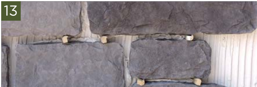
Stone application with joints
