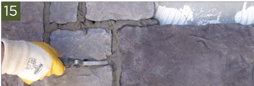
Stone application with joints
