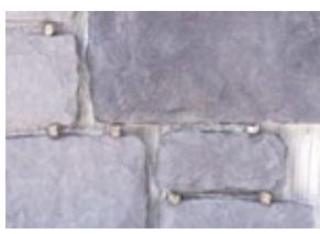
14 Installation of stones with joint: To stabilize the stones at the proper distance, small spacers should be used.
