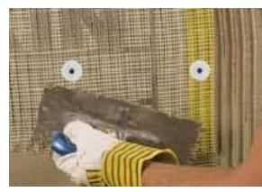
6 Apply the 1st base coating layer, the alkali resistant mesh, the anchors and the second layer of base coating.
