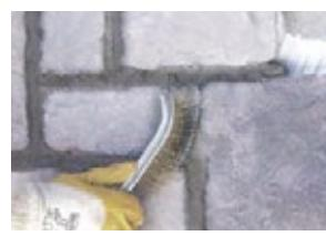
17 After approximately one hour brush off the mortar that lays on the stone surface with a hard plastic or soft wired brush.
