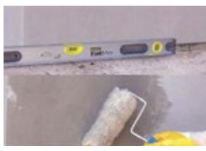
9 Clean the substrate from dust dirt and ensure that there are no weak areas. Apply the primer.
