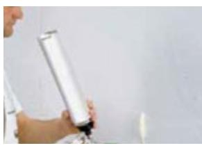
4 Seal all joints that exist between panels with low expansion polyurethane foam.
