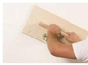
5 Grind installed panels to have smooth surface.
