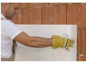
3 Apply the thermal insulation panels, (at least 24 hours idle time till the next step).
