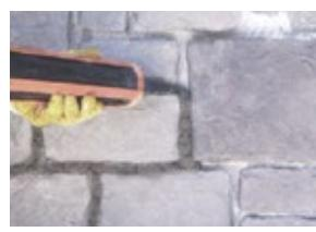
15 For grouting use a pastry bag or the special grouting gun. Apply the right quantity of mortar until the joint is filled.
