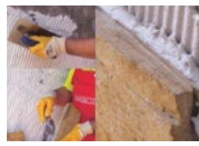
II Apply the adhesive on the installation surface and on the back surface of the stone.
