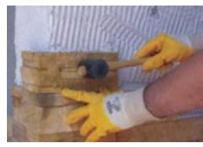
12 If installation includes corners, begin from the corner of the wall and continue the formation of the line using flat pieces. Use a rubber mallet to knock each stone piece.
